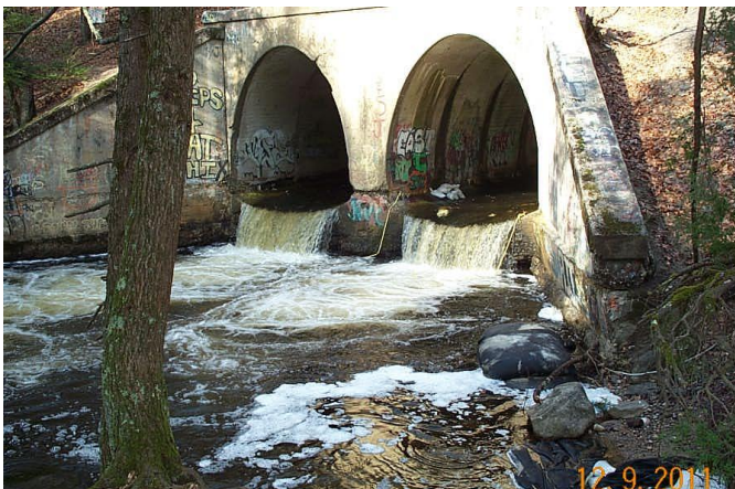
BEFORE: The Lyman Viaduct culvert at Dickinson Creek was a barrier to the migration of fish for over 50 years.
