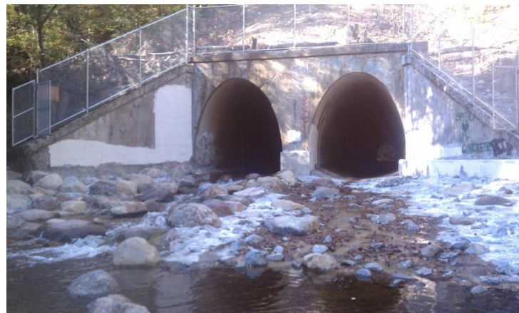
AFTER: The repair of the culvert included a rock ramp fishway on the west side, through which all low flows are diverted.
